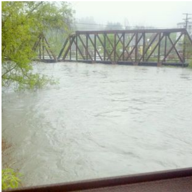
3 4 Figure 7: May 2011 Flooding on Memorial Drive Bridge. City of Montpelier Public Works
