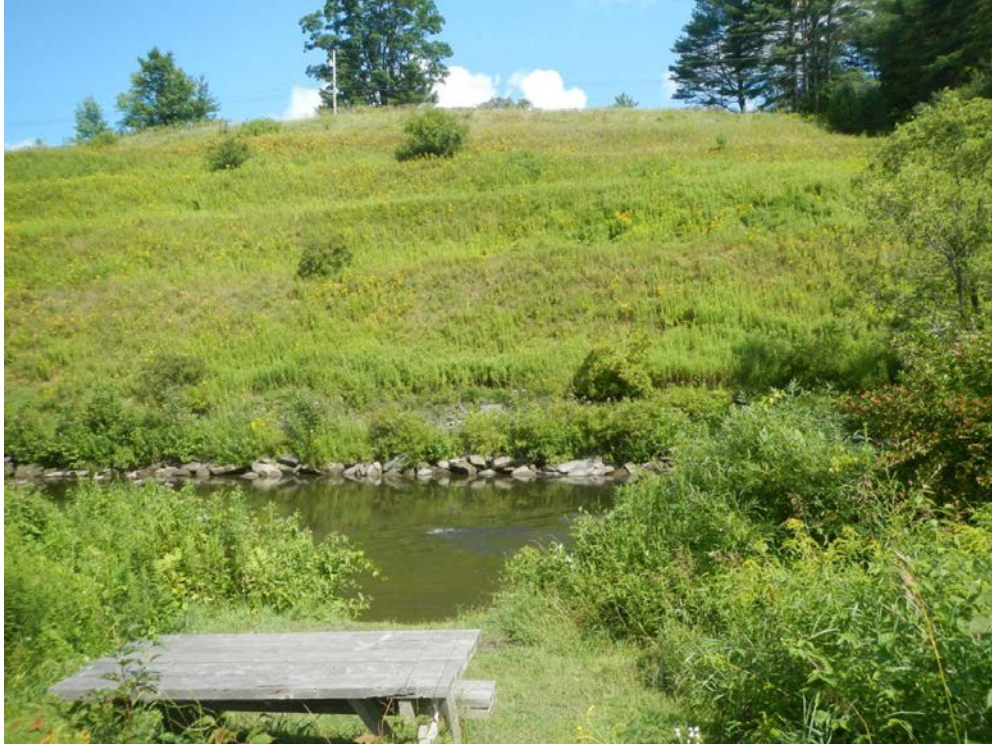
Photograph 27: Picnic table and hill supporting Gould Hill Road, taken from North Branch Nature Center
