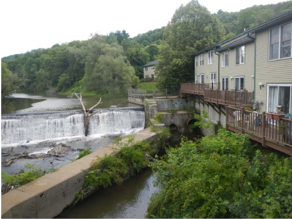
Photograph 17: Dam above Vine Street footbridge on the North Branch of the Winooski
